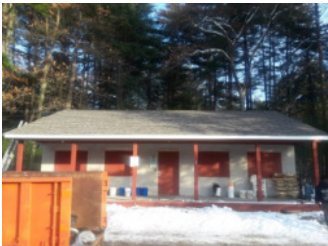
New Shooters Den Roof (Good work completed by Andy Woods)
